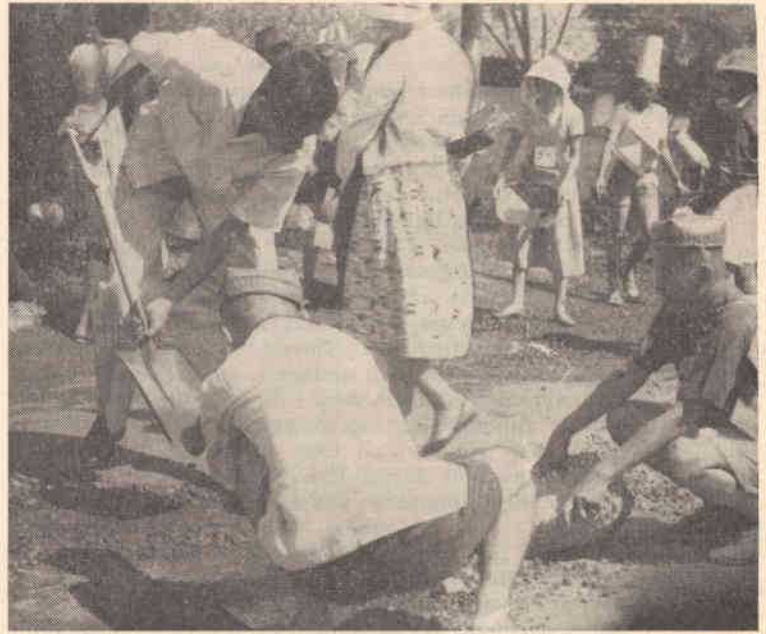
...while the men repair the roads
